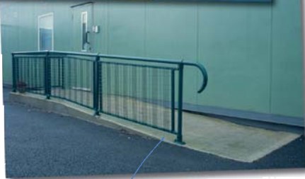
note accessible entrance
